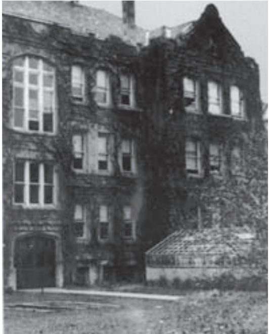
“Wylie Hall. Kinsey’s ‘laboratory’ took up most of the basement from 1950 onwards.” (Caption and photo taken from Gathorne-Hardy’s Sex, the Measure of All Things .)
